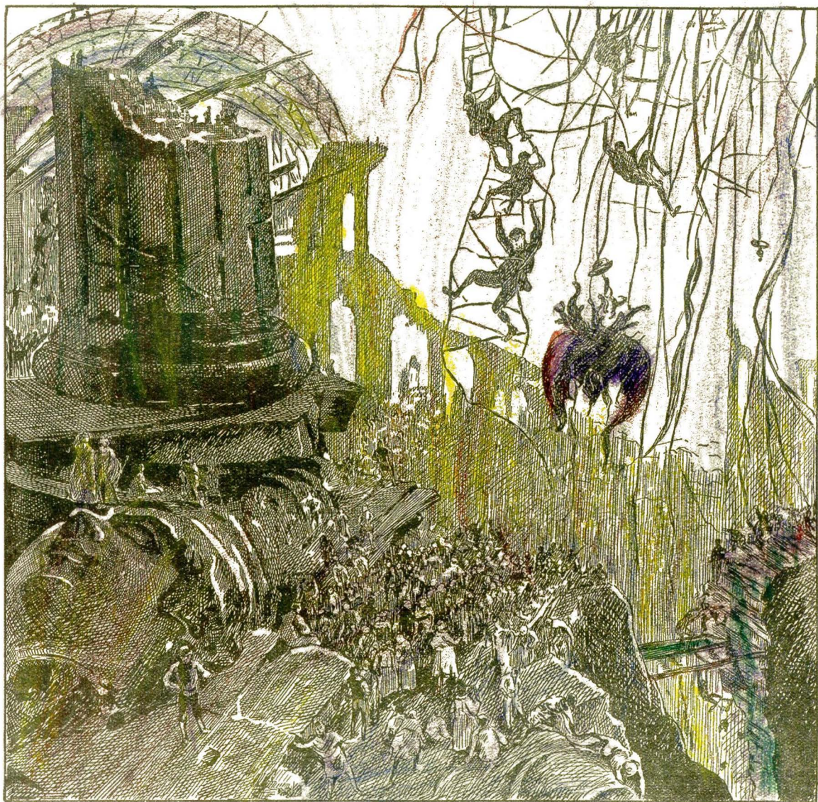
Vast masses of twisted cable dropped like tangled sea-weed.
